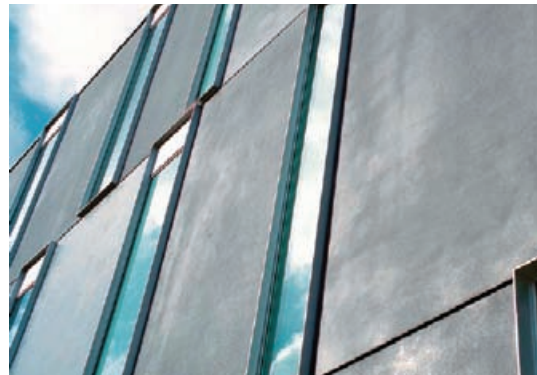
PRECAST CONCRETE: M2
